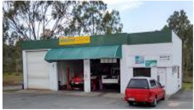
Round House Mechanical workshop at North Maclean North
