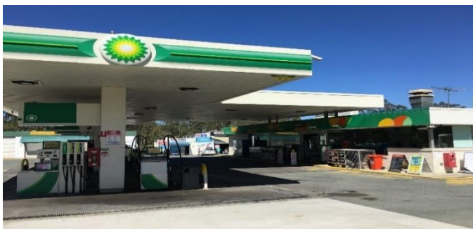
BP Service Station North Maclean & Regents Park
