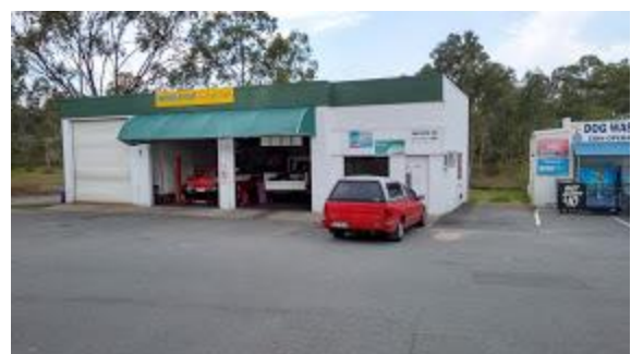
Round House Mechanical workshop at North Maclean
