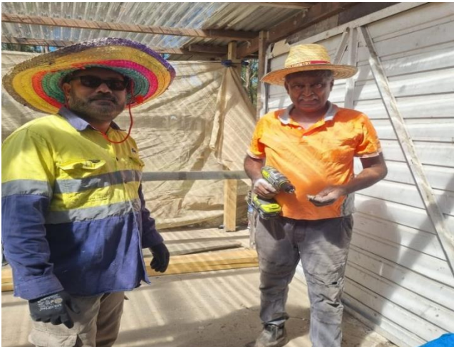
Board members Dhirendra Singh and Braham Deo helping in the cleaning and fixing the old shed.
