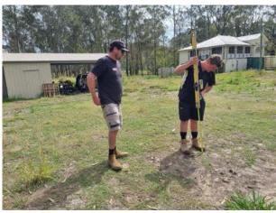
Luke (Plumber) and Teejay (Concreter) measuring the pad height to meet the Council requirements. They have been working together to re-schedule the earthworks and concreting as soon the weather permits.
