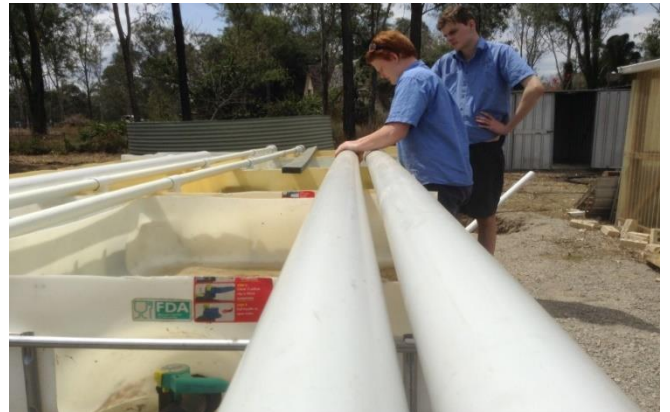
Caleb Sutcliffe (Cert II qualified plumber) assisting Nick with Plumbing
