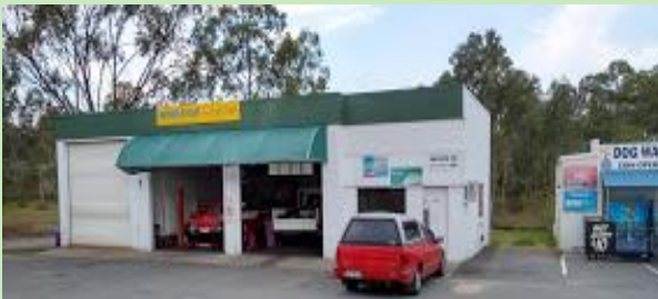
Round House Mechanical workshop at North Maclean North Maclean Produce Shop
