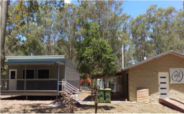
Left: Fully air-conditioned classroom Right: Our refurbished Administration Building
