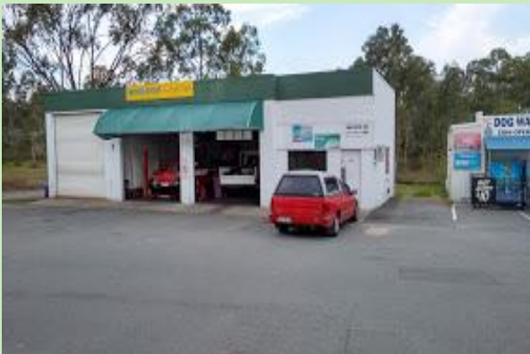
Round House Mechanical workshop at North Maclean North Maclean Produce Shop
